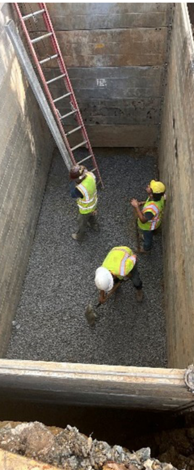
Installation of electrical manhole structure on Feeder 15001 at Kennedy Street
