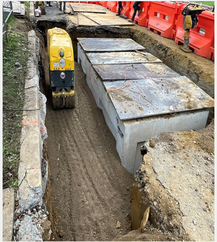
Installation of electrical manhole structure on Feeder 15001 at Kennedy Street
