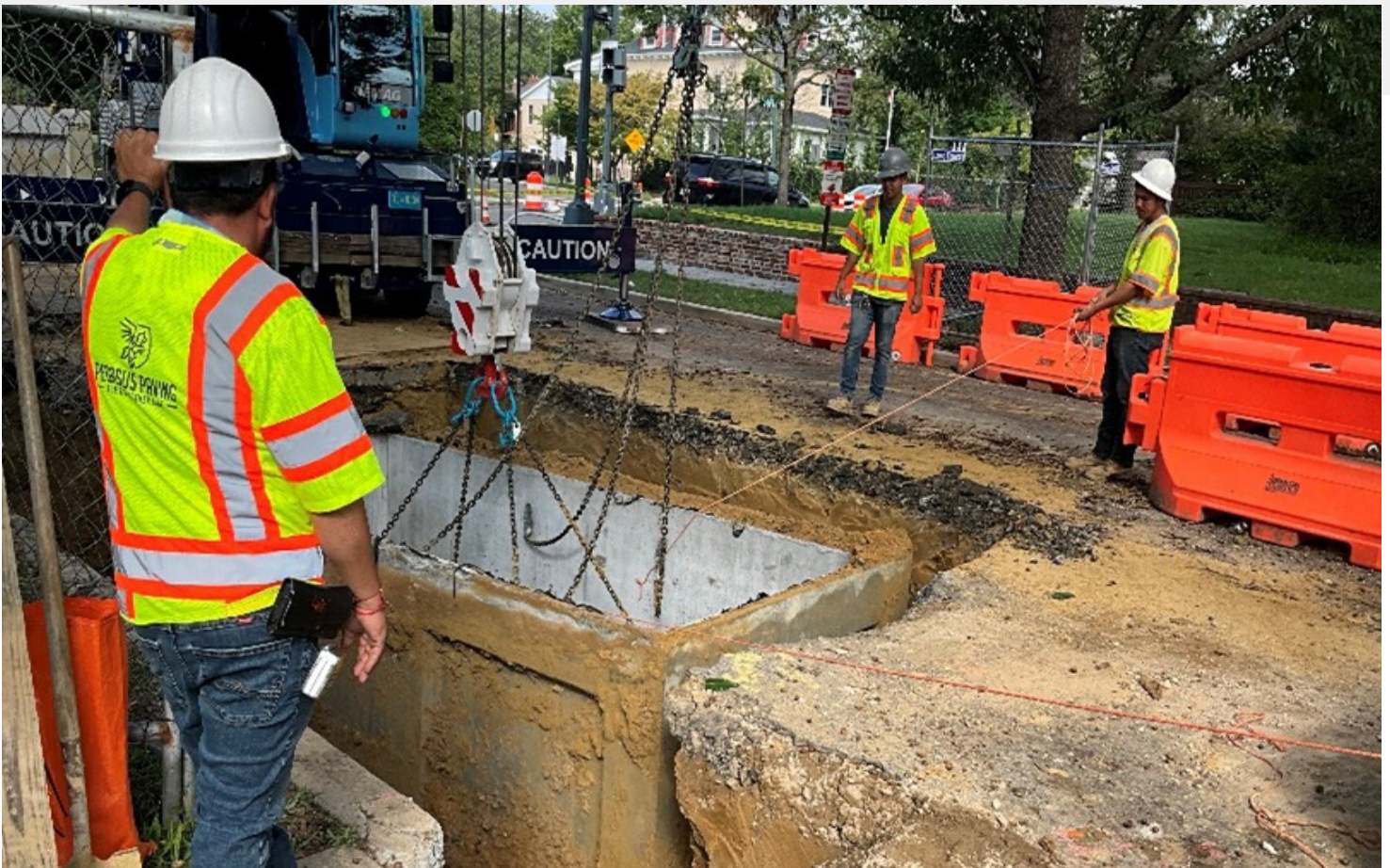
Installation of electrical manhole structure on Feeder 15001 at Kennedy Street
