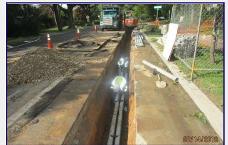
Conduit is laid
