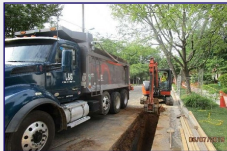
Trench is excavated
