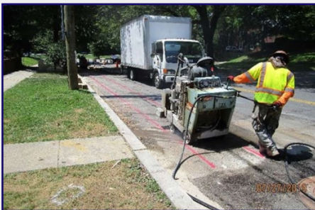
Marked & saw cut
